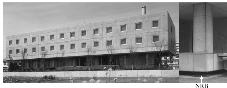
Figure 1 Appearance of the building
