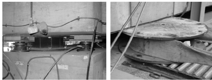
Figure 4 The view of replacing a rubber bearing (2008)
