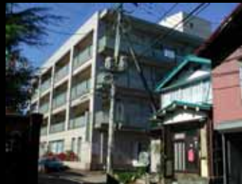
South-east view, no external damage
