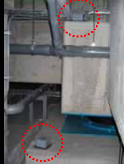
Motion sensor above and below Isolator
