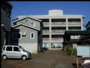
South view, no external damage
